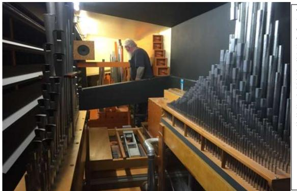
This is the workings of the church's pipe organ before the metal and wooden pipes and sound boxes were removed the first part of June to take to Morel Organ Works to be repaired, cleaned, rewired, and returned.
